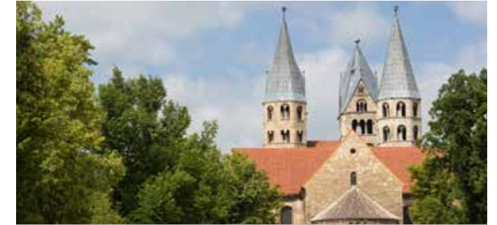
Ceramic Membrane and Module Production Halberstadt, Germany
